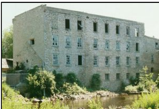
c. 1970 Demolition begins on the Watchorn Woollen Mill built originally by Stephen Merrick in 1848
